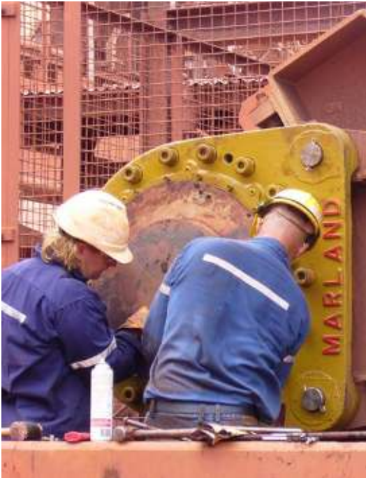
Marland Backstop Model BC-375MA being installed at taconite mining operation
